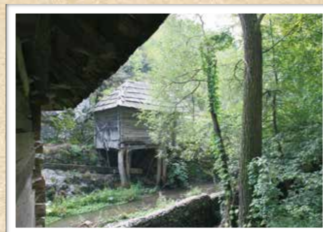
Eftimie Murgu Village – The Little indomitable” Mill– 20th century LMI (List of Historic Monuments) CS-II-m-A-11112.07 / Sat Eftimie Murgu – Moara „Îndărătnica Mică” – sec. XX / LMI (Lista Monumentelor Istorice) CS-II-m-A-11112.07 / Selo Eftimie Murgu – Vodenica „Îndărătnica Mică” – XX vek / SSK (Spisak spomenika kulture) CS-II-m-A-11112.07
