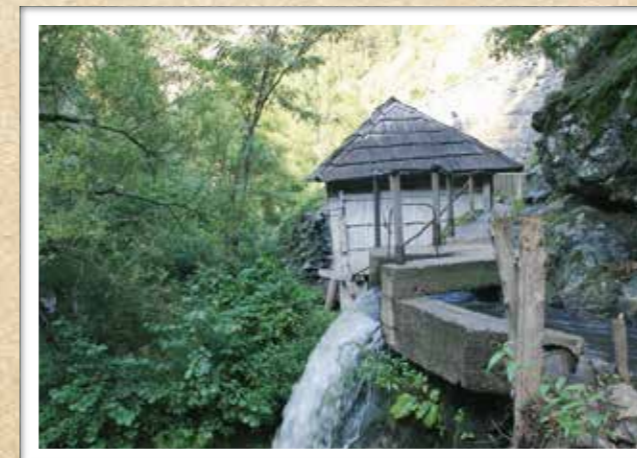
Eftimie Murgu Village–TRĂILOANEA Mill (rear view) – 20th century LMI (List of Historic Monuments) CS-II-m-A-11112.10 / Sat Eftimie Murgu – Moara Trăiloanea (vedere din spate) – sec. XX / LMI (Lista Monumentelor Istorice) CS-II-m-A-11112.10 / Selo Eftimie Murgu – Vodenica TRĂILOANEA (pogled s bočne strane) – XX vek / SSK (Spisak spomenika kulture) CS-II-m-A-11112.10
